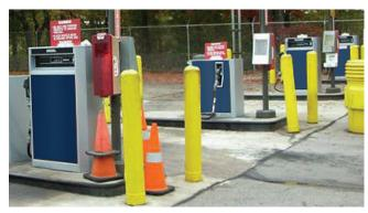
All remote dispensers include a satellite connection as standard so that they can be piped to an opposing satellite dispenser for the convenient fueling of truck saddle tanks or vehicles positioned with their tank on the opposite side.
